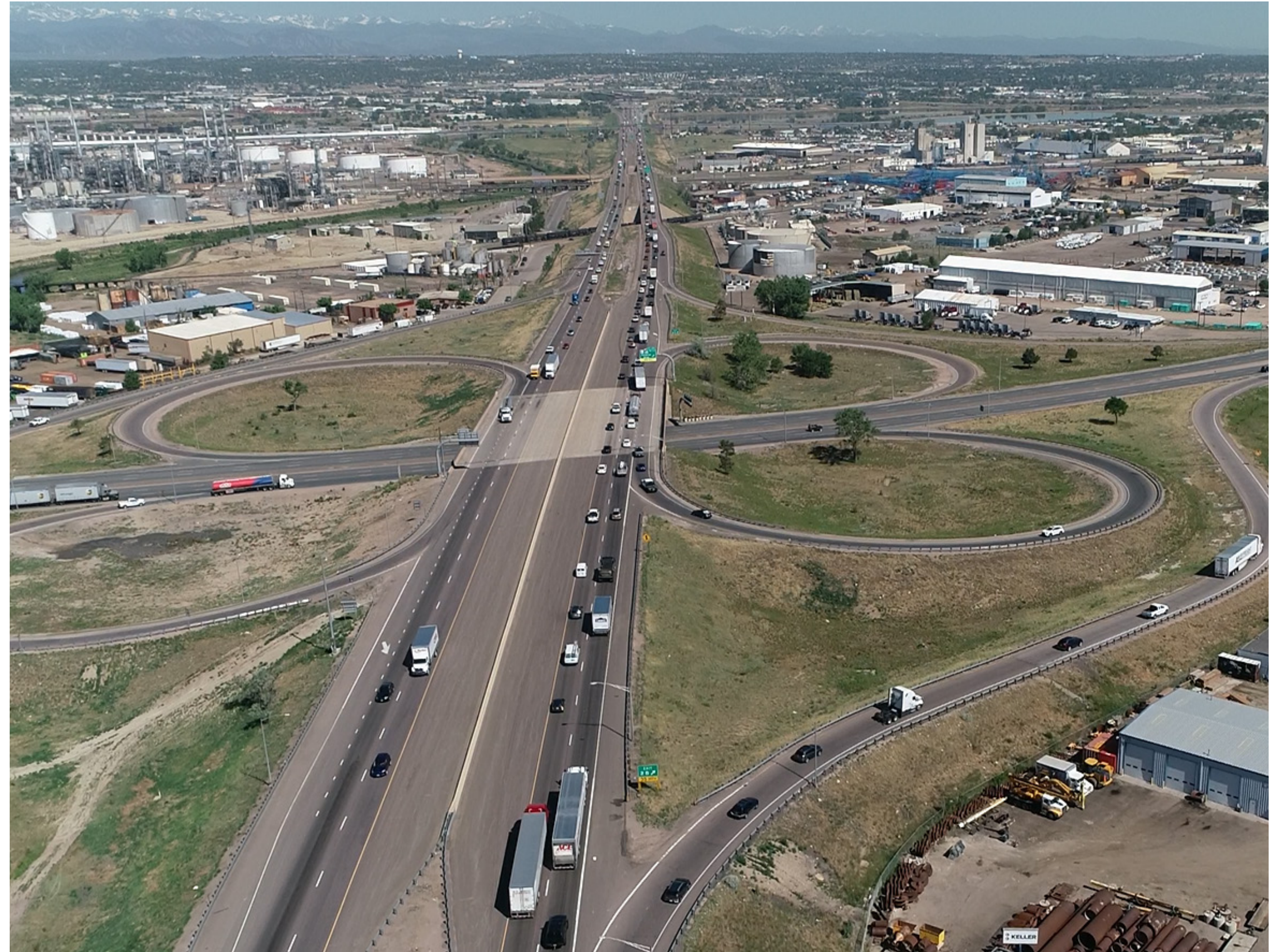
I-270 looking west from Vasquez Boulevard interchange
